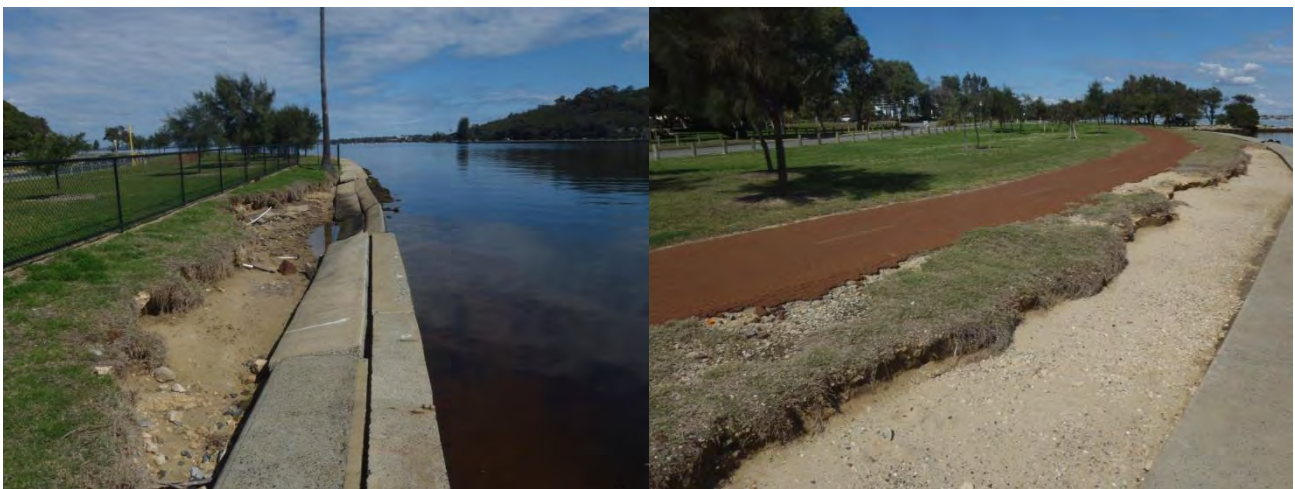
Plate 4: Erosion damage along Narrows foreshore a) to river walling and b) threatening footpath
