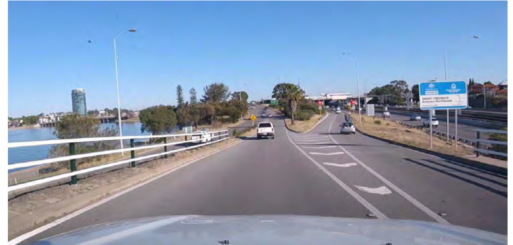
Figure 22 Screenshot of in-car footage - Manning Road on-ramp to Freeway early
