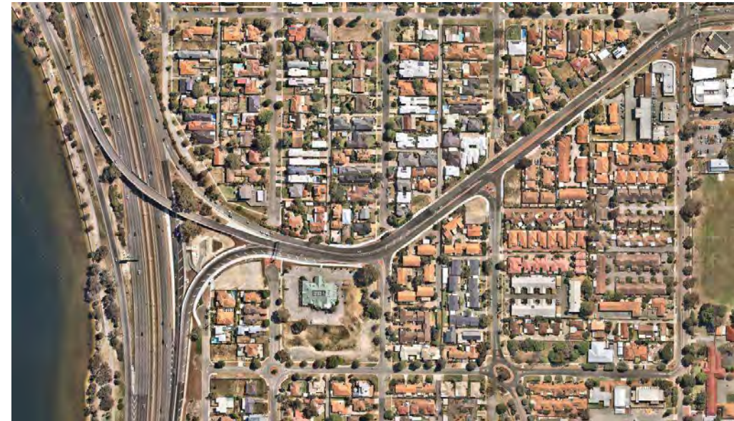
Figure 83 Aerial image of new southbound ramp (source: Nearmap)
