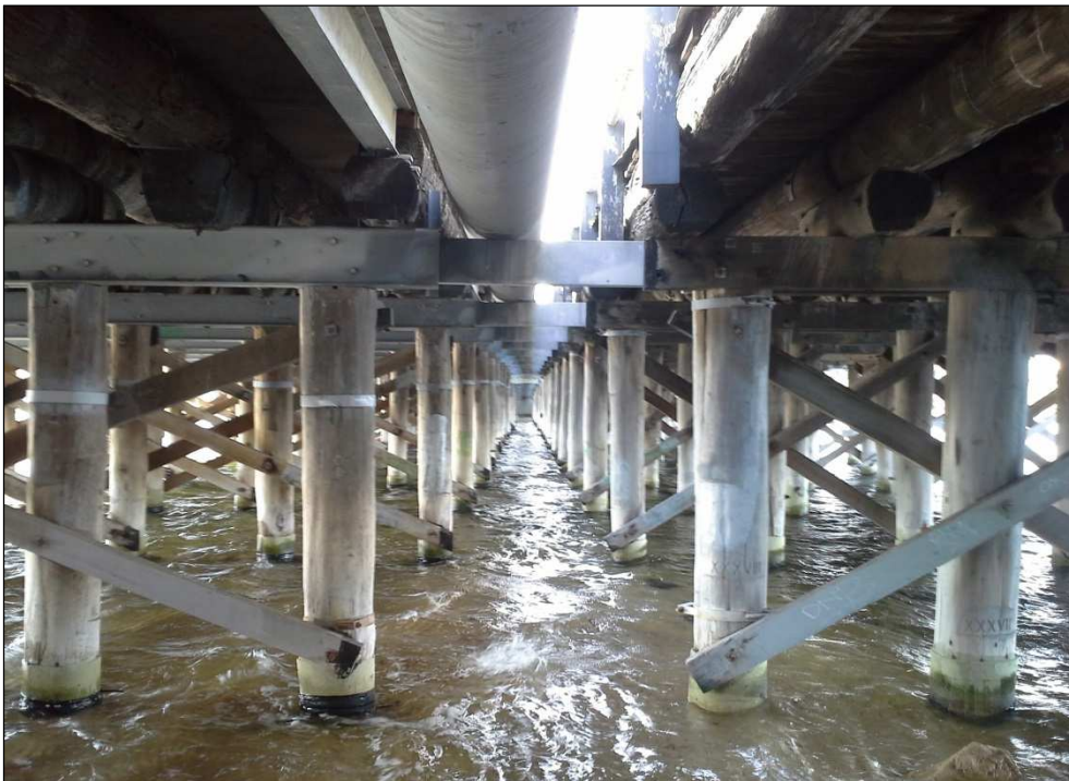
A view of the under-structure of the Canning Bridge at the central gap between the 1938 (left) and 1958 (right) bridges. (Gina Fraser, City of South Perth, 1 June 2015)
