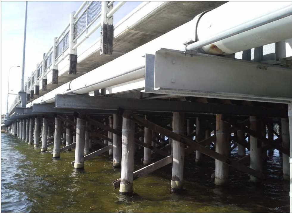
Close-up view of Canning Bridge No. 4 (1938) from north-western side showing its form and structure, including service conduits fixed along the side of the Bridge. (Gina Fraser, City of South Perth, 1 June 2015)
