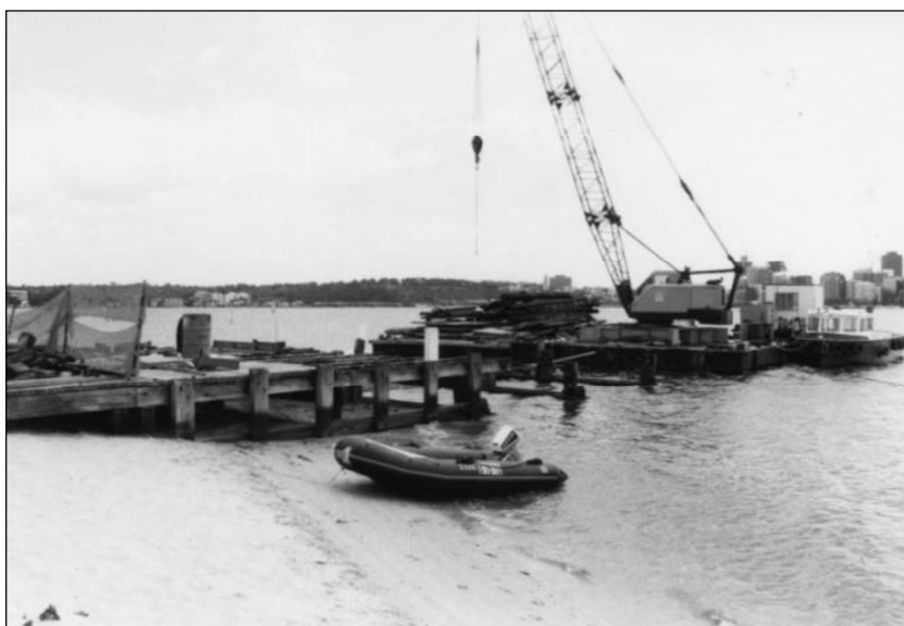
Crane on demolition barge in the process of demolishing the Coode Street Jetty, 1990. (Picture South Perth Photograph Collection)
