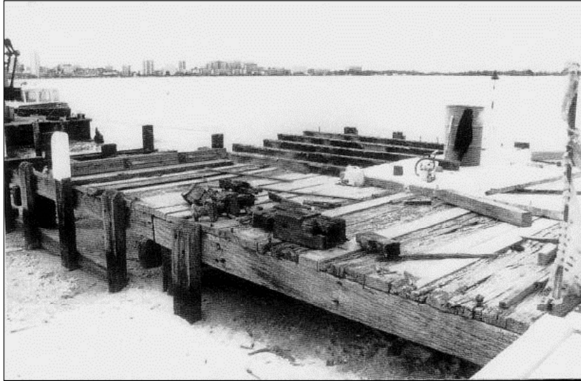
During the demolition and rebuilding of the Coode Street Jetty, 1990.
