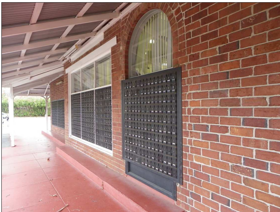
Verandah containing the former doorway opening on the Mends Street elevation. The location of the opening is identified by a round arch formed with red brick voussoirs. (Gina Fraser, City of South Perth, 2015)
