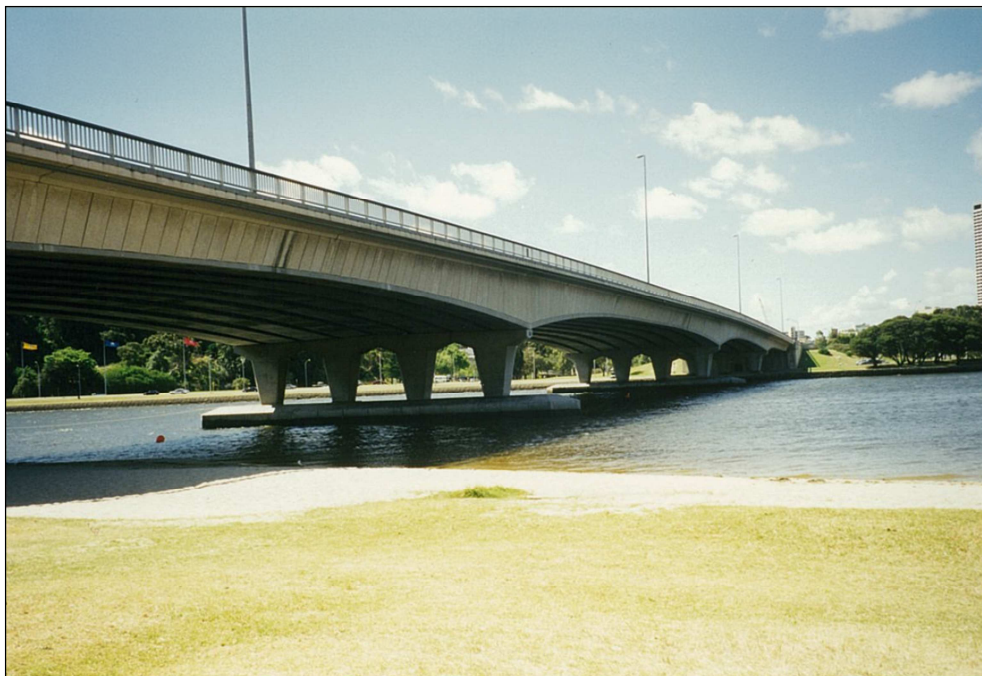
The original Narrows Bridge which was constructed in 1959. (Heritage Today, 1999)
