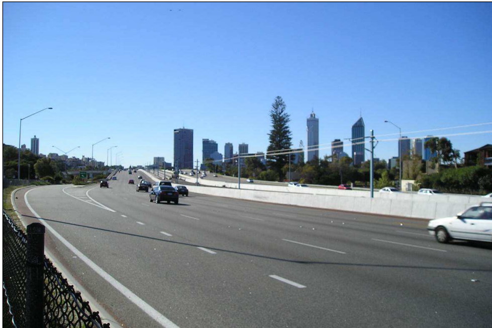
The Narrows Bridge comprising two traffic bridges with a central railway bridge. (Gina Fraser, City of South Perth, June 2007)
