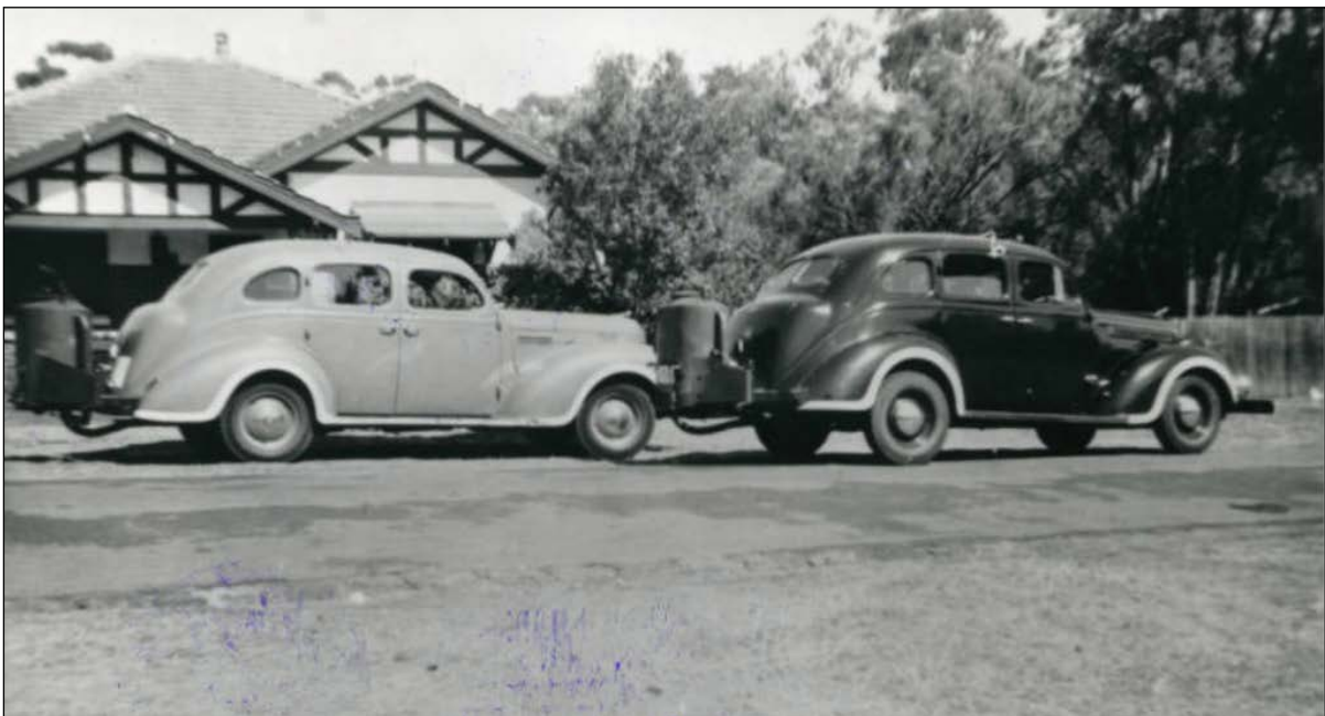
Figure 20 Taxis with gas converters, necessary owing to fuel shortages in World War II, 1943.
