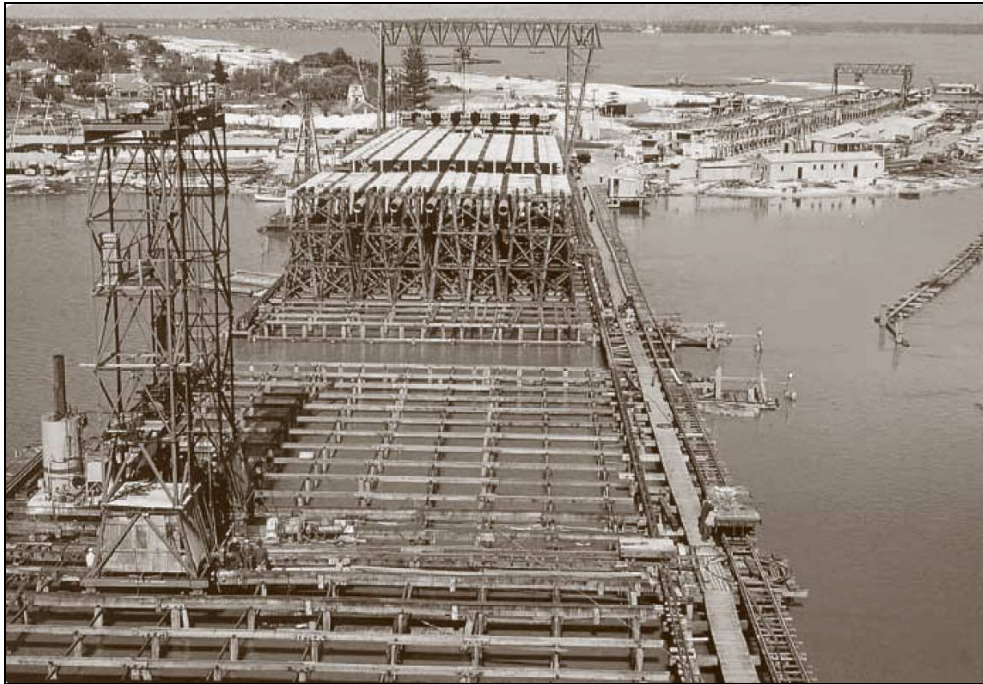
Narrows Bridge under construction c1958.
