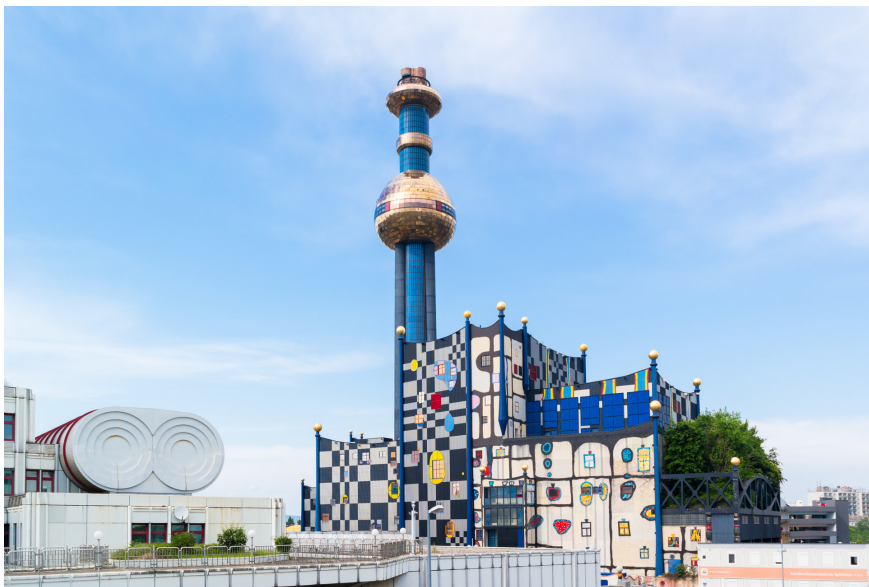
SPITTELAU EFW PLANT (VIENNA) - SUCCESSFULLY OPERATING SINCE 1971
