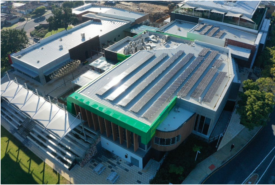
Figure 7: Manning hub solar PV system
